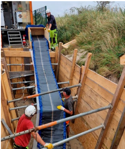
The compact transport dimensions of the Alphaliner facilitated the pipe repair in the UNESCO World Heritage Site
