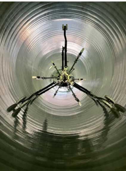
Piece by piece, the UV system moves through the fitted liner and cures it
