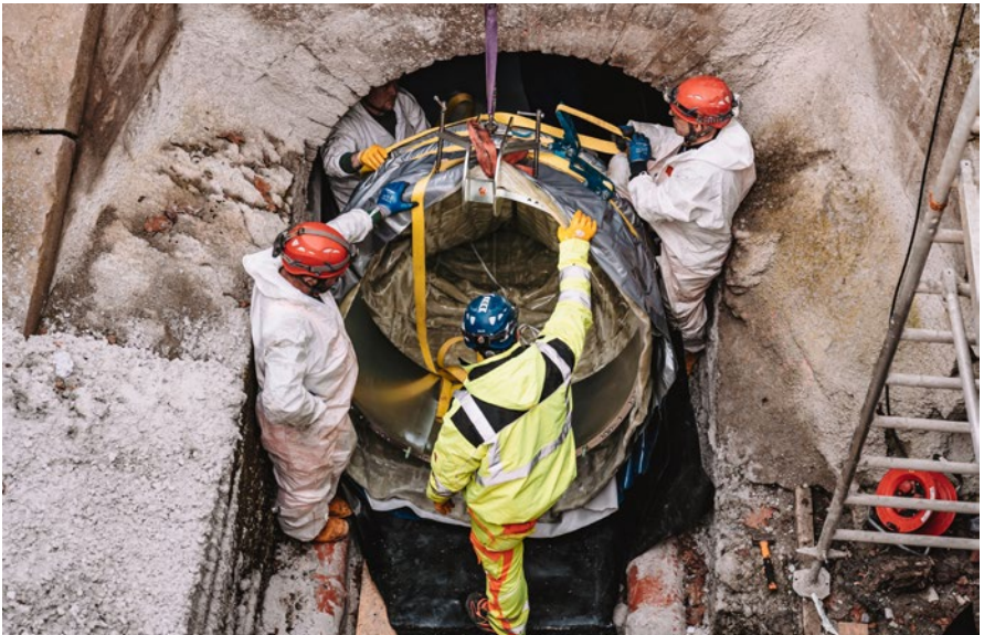
Every liner installation is a team effort by experts
